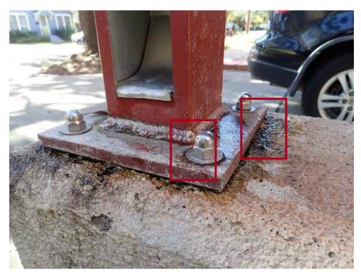
25 Latent moisture and corrosion at base of column
