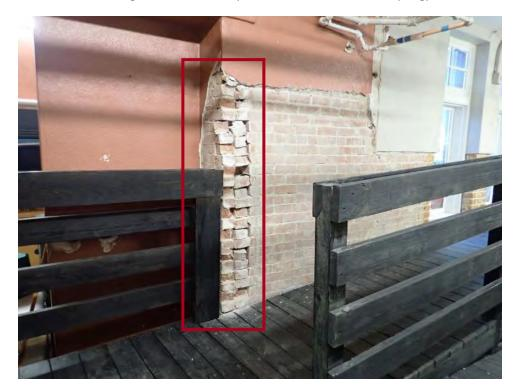
O6 Loose and missing bricks in an intersecting brick wall
