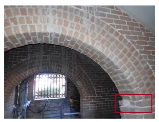
O5 Missing bricks and severely deteriorated mortar at the springpoint
