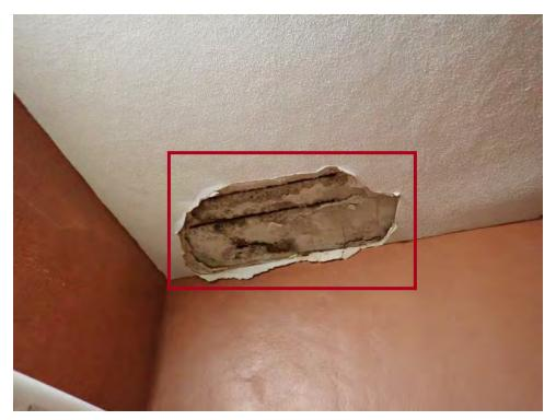
${\color{red}08} \qquad \qquad \text{Overhead spall in the interior storage room under the main entrance}$
