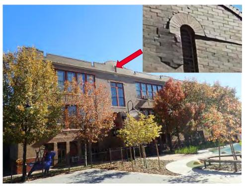
West elevation, the area with bulged bricks is enlarged
