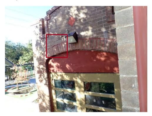
11 Stair step cracking above the arch
