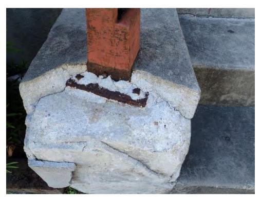
17 Spalled concrete door stop at Southwest Corner
