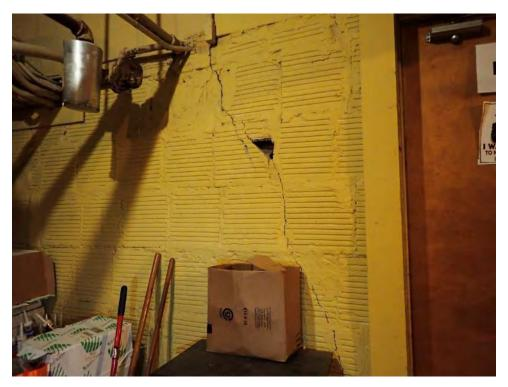
21 Cracking of clay infill tiles
