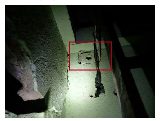
22 Missing roof access ladder support
