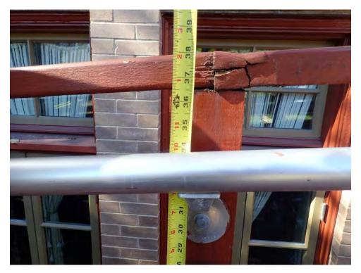
15 Deteriorated wood handrail at East Entrance3
