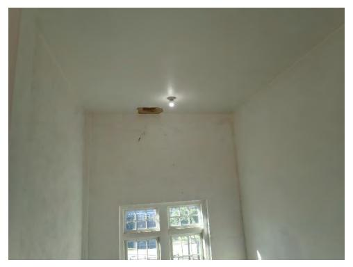
Overhead spall in South Stairway
