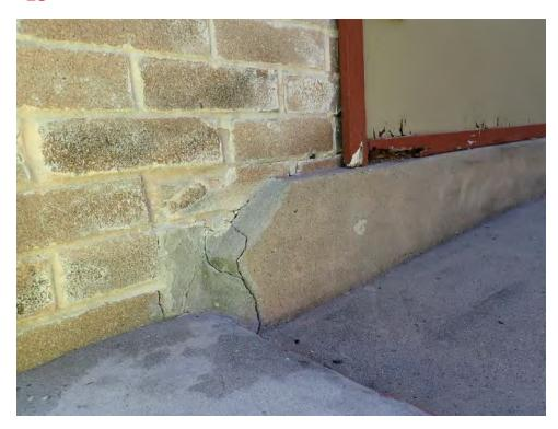
16 Spalling curb on North side of East Entrance
