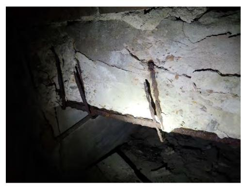
O3 Exposed corroded rebar on back entrance to ventilation shaft
