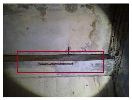
O7 Spalling overhead slab under main entrance
