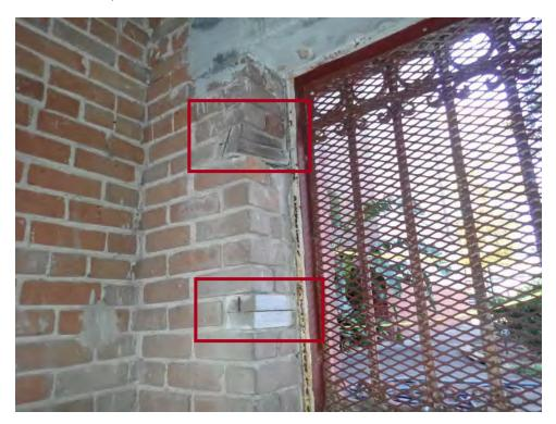
O4 Missing bricks at gate under bearing end of concrete beam
