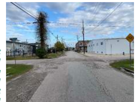
Top left: Silver Street north of Dart Street, looking north
