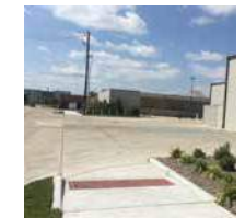
Accessible Ramp and Traversable Sidewalk
