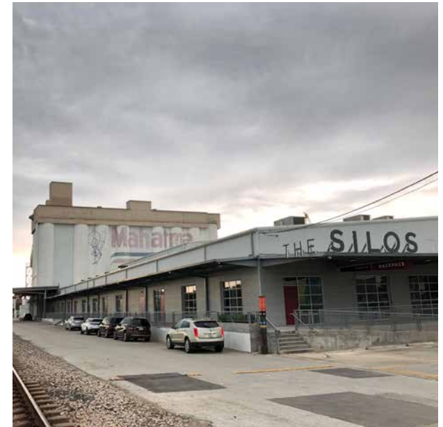
The Silos at Sawyer Yards
