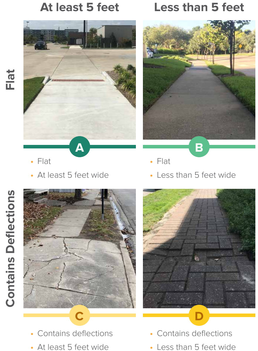
Figure 3. Sidewalk Condition Matrix
