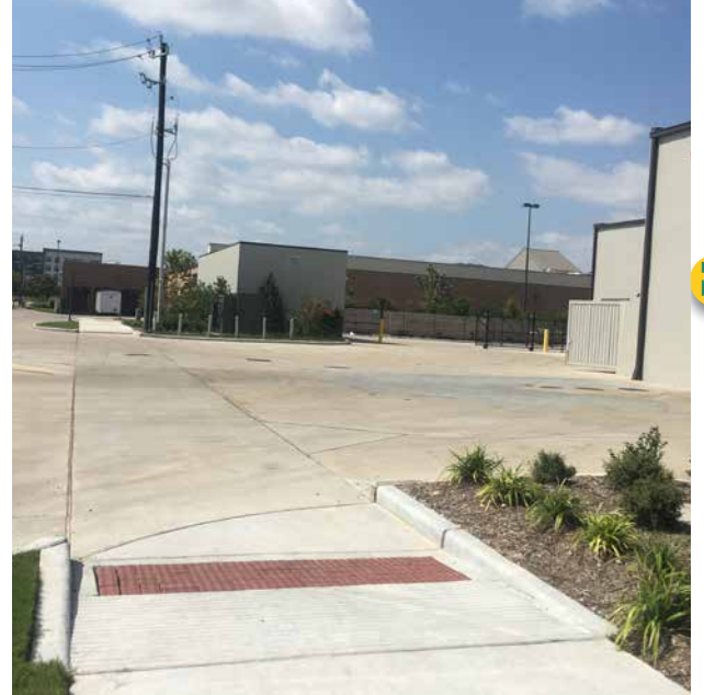
Newly Built Ramp to ADA Standards
